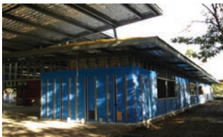
Palm Beach State School - During Construction
